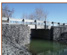
4.1 m Concrete Box Culvert Built: 2014
