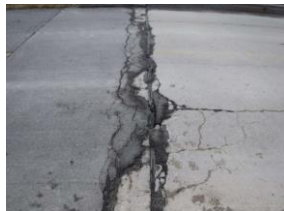
South Expansion Joint
