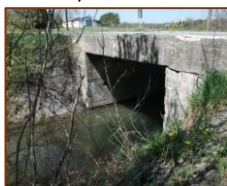
3.7 m Open Footing Culvert Built: 1944 (age: 71 years)
