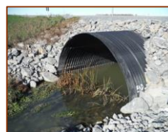
3.5 m CSP Culvert Built: 2013
