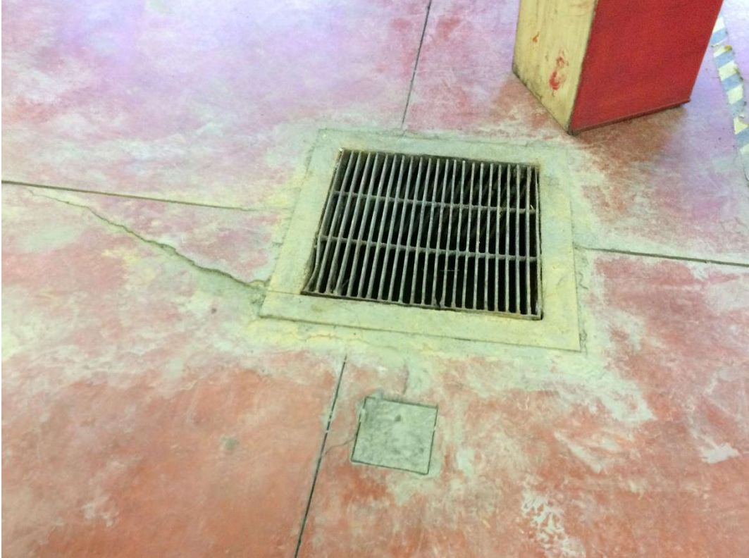
Photo 14. Drain and slab cracks
