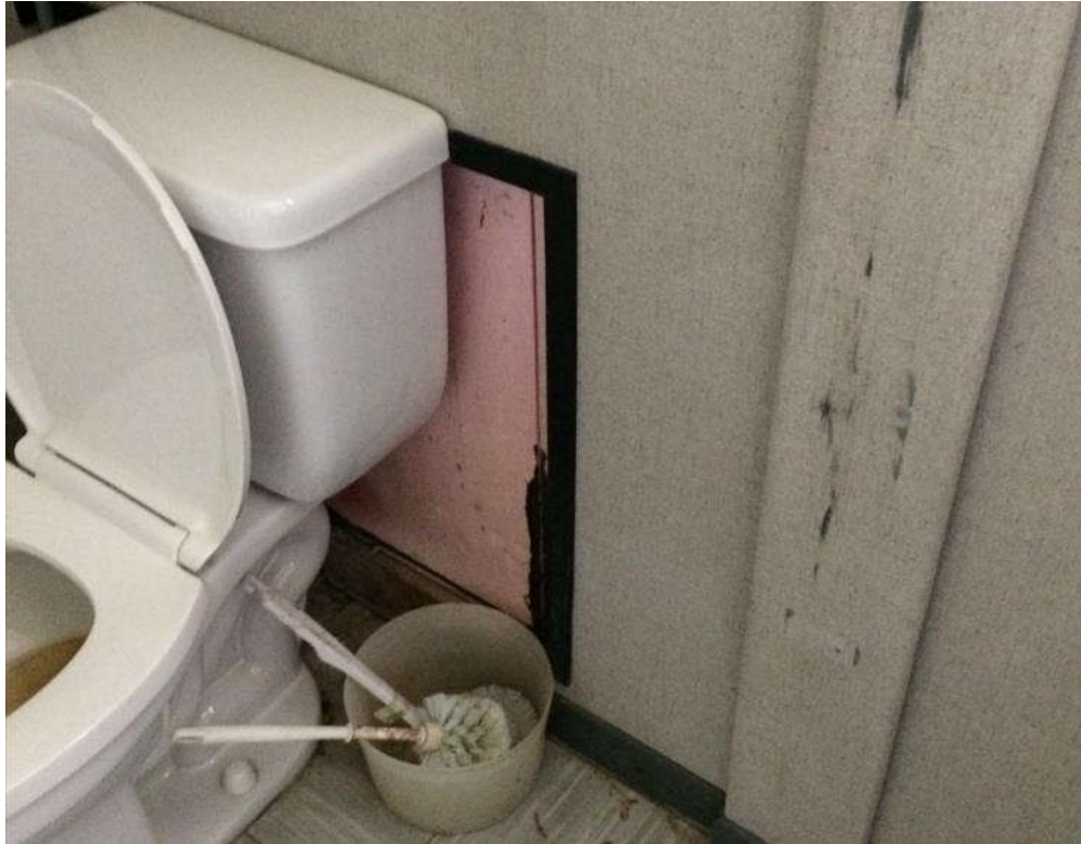
Photo 16. Insulation in washroom
