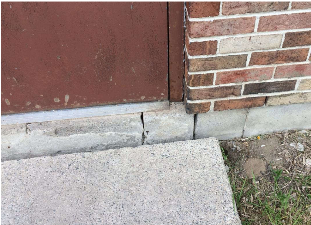
Photo 9. Head joints crumbled
