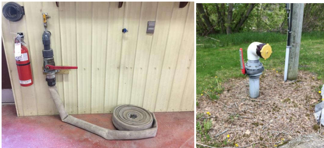
Photo 4. Interior and Exterior Fire Hydrants
