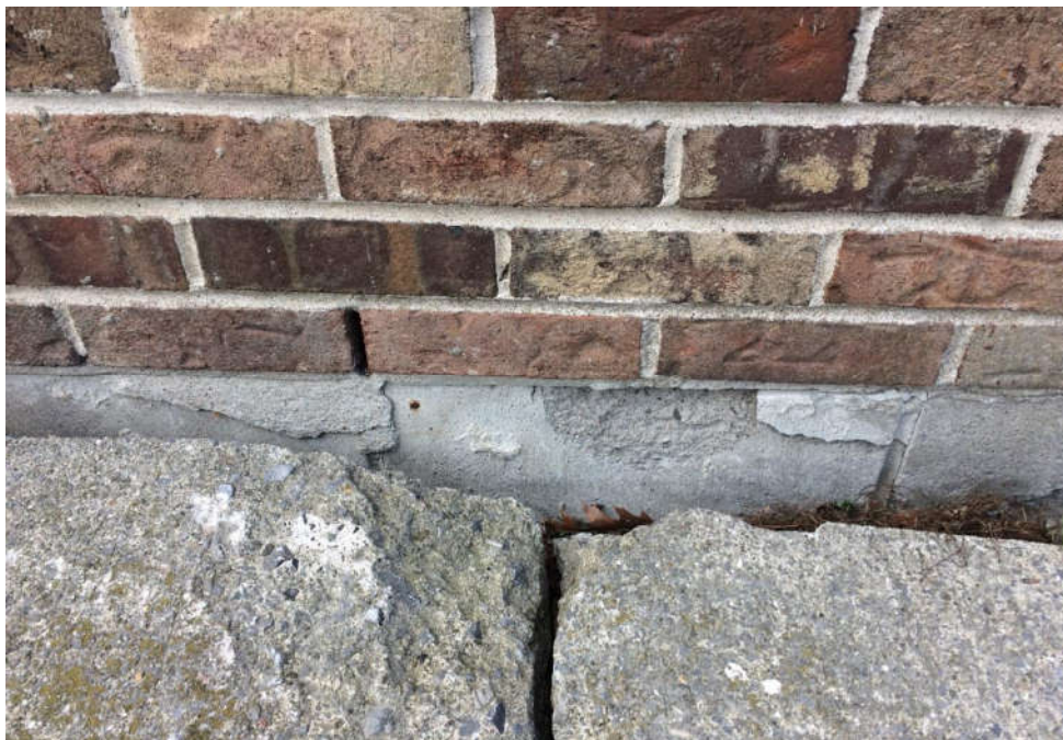
Photo 7. Foundation parging and block
