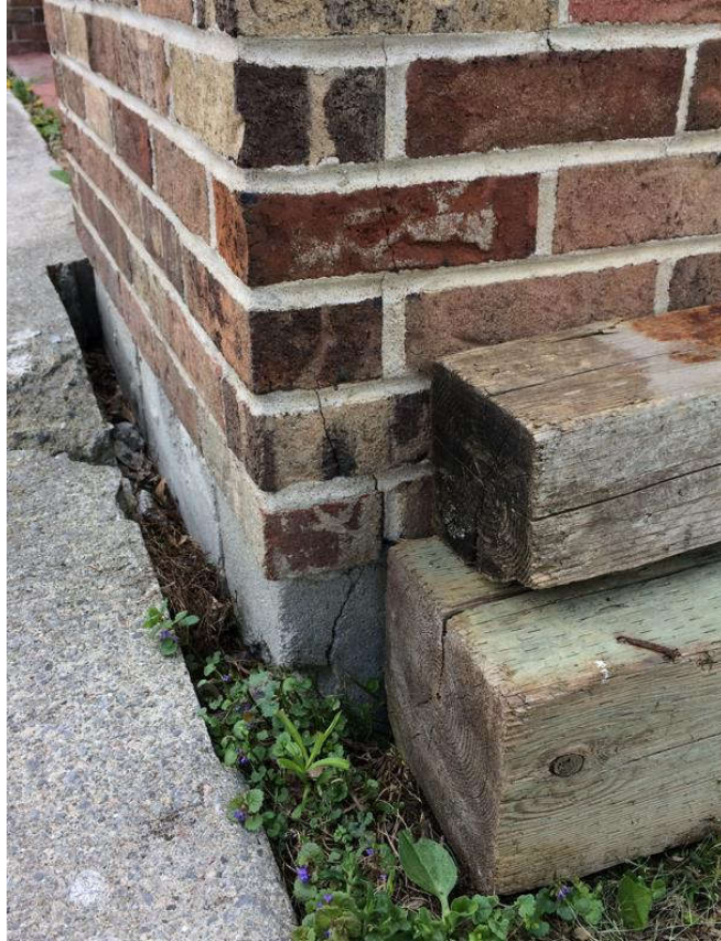
Photo 10. Cracking in foundation and wall facade
