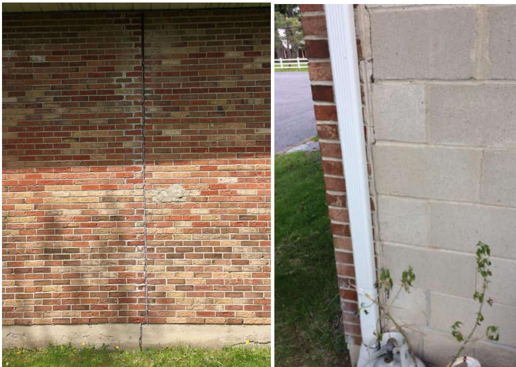
Photo 11. Expansion joints separation
