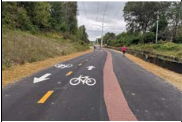
Example of a dual trail system (W&OD Trail) in Arlington, VA. The central pavers are permeable while also visually separating the two user groups.
