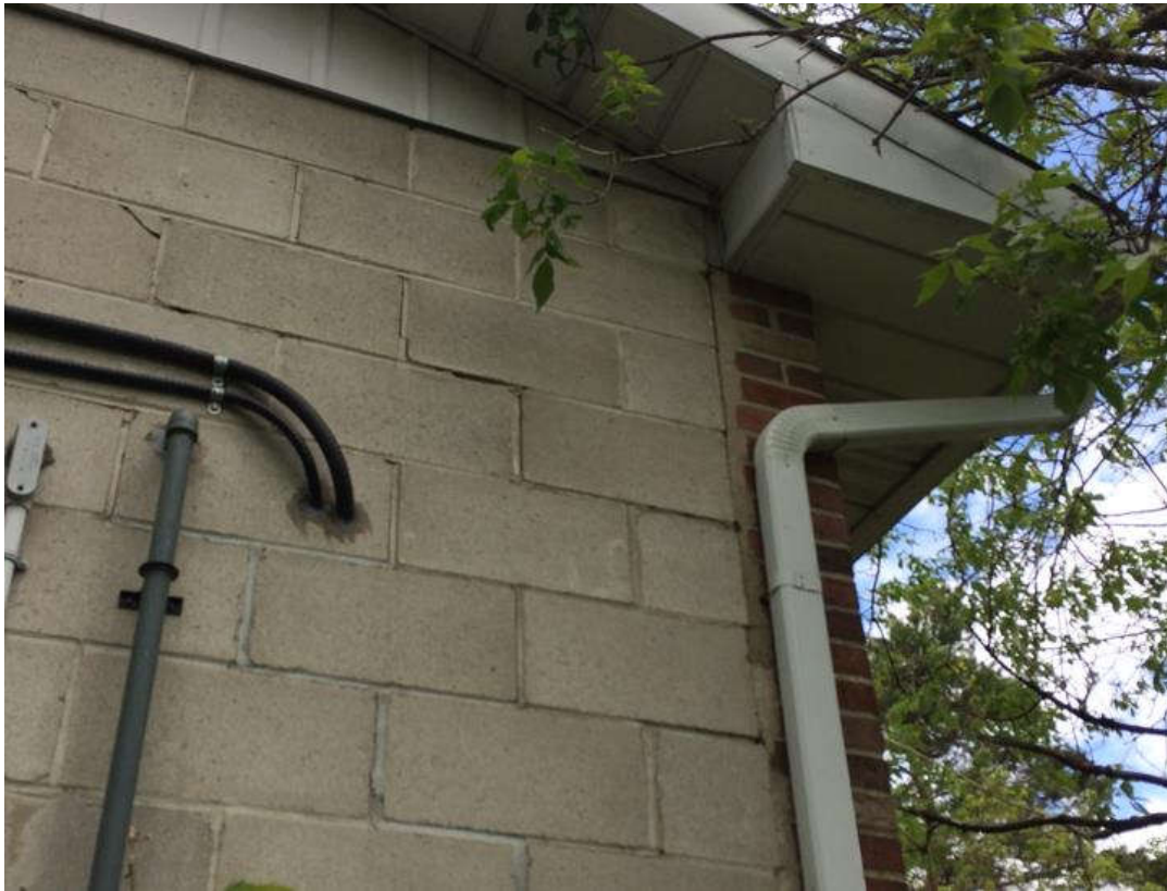
Photo 12. Diagonal cracking at south elevation
