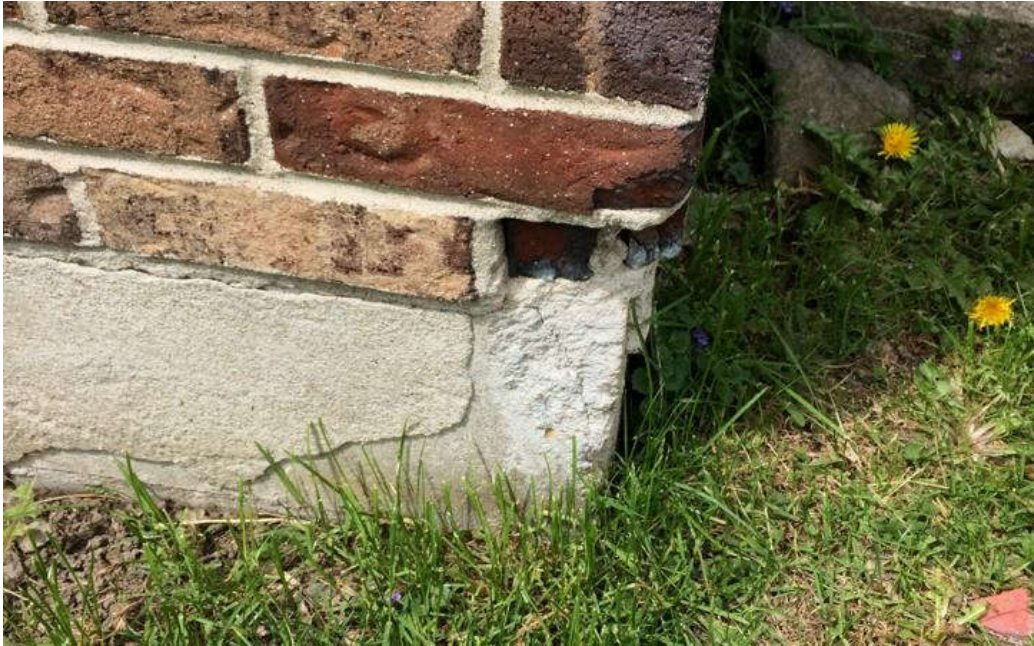
Photo 8. Foundation parging and spalling of block
