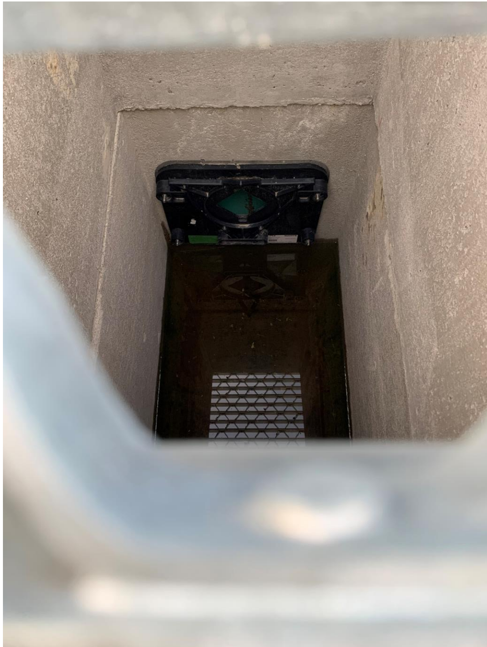
Photograph 16: SWM Facility Outlet Structure ICD (to be relocated)
