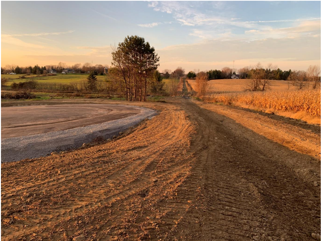
Photograph 11: Berm between East End of River Road and East Ditch (Separating Drainage Areas)
