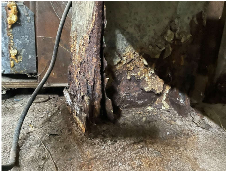
Photo 1: Workshop Column Corrosion
